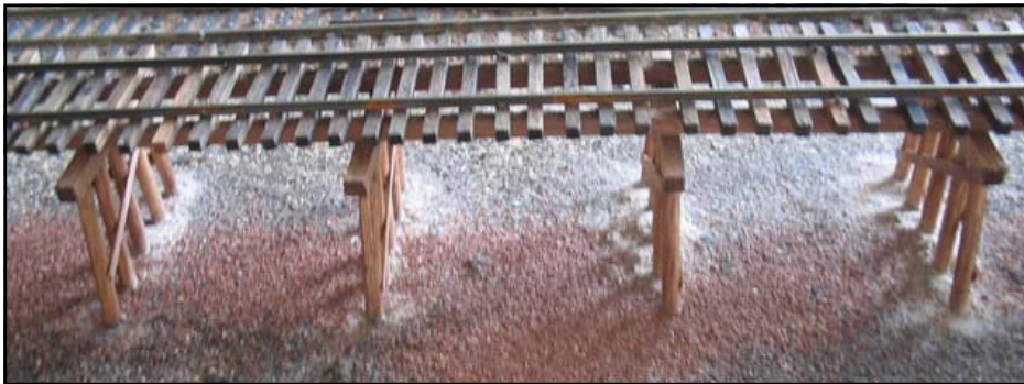
Fig. 6 Above: This photo depicts the first placement of the completed elevated wood trestle, less track. The bents, stringers and ties are all in place. The bents do not rest even with the surface at this stage but when glued in place and held with scenic material the whole structure will appear to be built into the topsoil.
