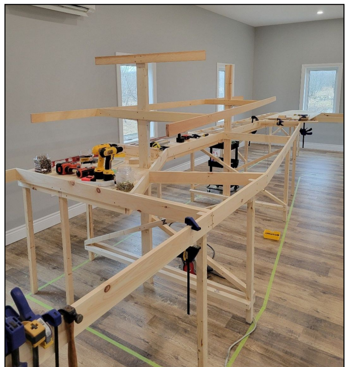
Photo Above: March 27, 2024: The progress on the benchwork continues with this photo showing the relative height of each level as well as the valance height.
