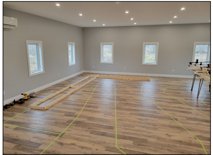
Photo Above: March 16, 2024: The first portion of benchwork started.
